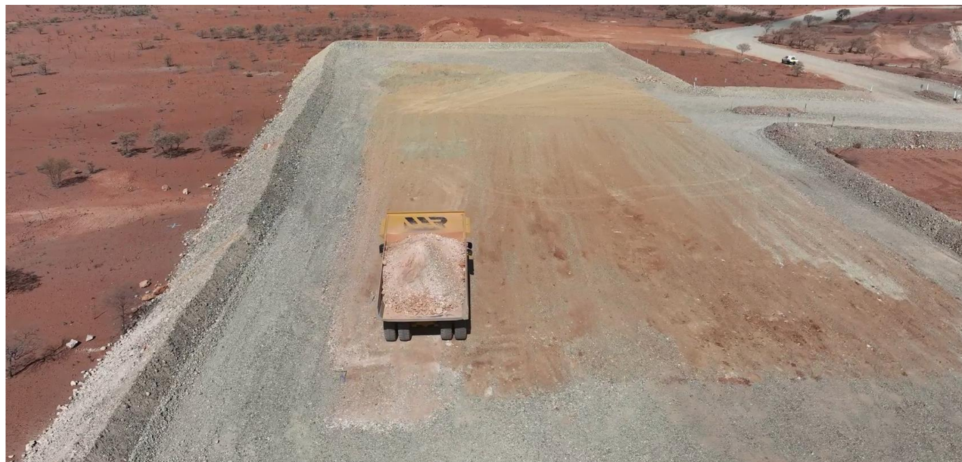
Figure 1 – Mineralised material being stockpiled on ROM pad at Tumblegum South Gold Project site
